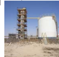
PM Surge tank & Gas Boot, Harouge Oil Operations
