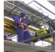
Construction of Workshops
