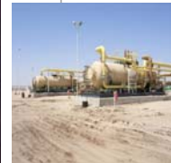
Repair and maintenance of Separators at Station 7, Veaba Oil Operations
